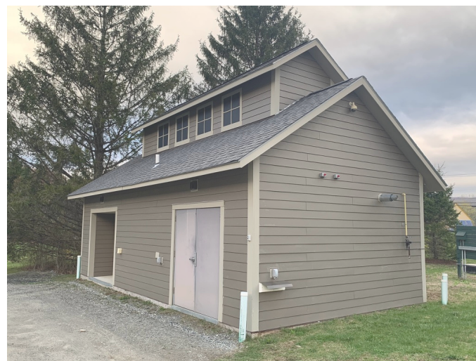
Photo: Control building, Waitsfield
