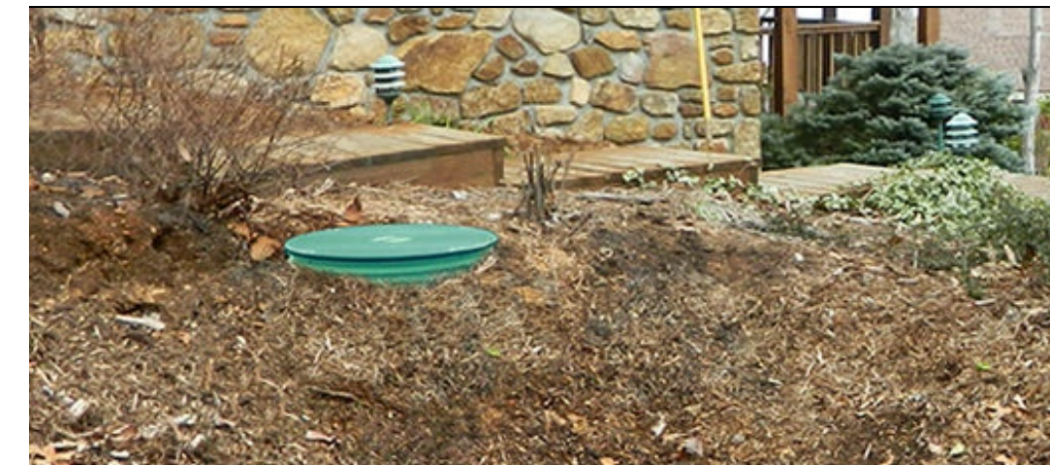
Photo: Typical septic tank lid
